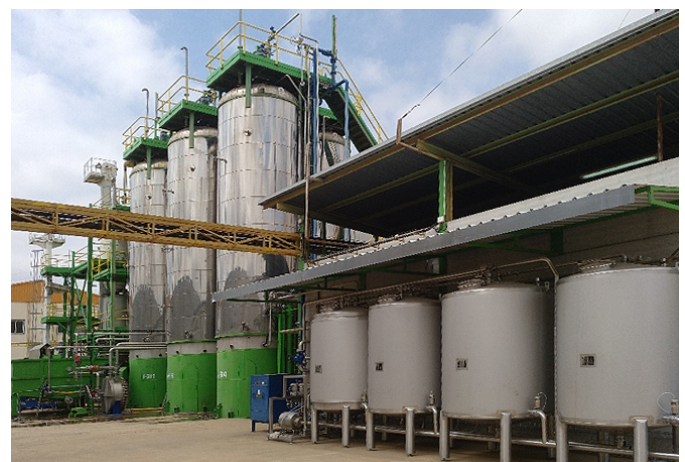
Figure 2: IMECAL facilities related to the PERSEO Bioethanol® plant where conversion of biowaste to bioethanol and bioethylene takes place at the demonstration-scale.
