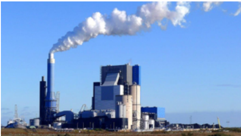
Coal-fired Rotterdam power plant into a biomass-fired heat and power plant (photo by Engie).
