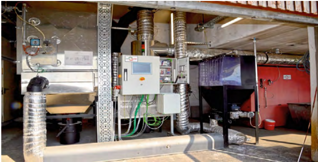
Figure 3: Field installation for the demonstration of the combined emission reduction on a biogenic residues combustion plant (© Karin Wilck)
